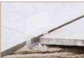
USE WITH "+" LAYOUT BOTH ON TILES INTERSECTIONS AND SIDES
